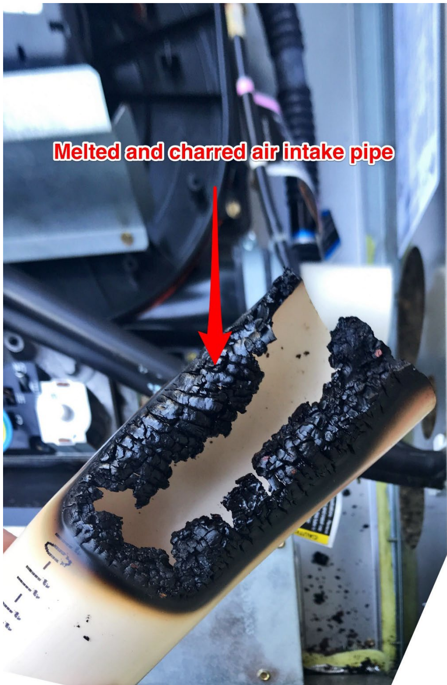
Image 5 – Air inlet pipe removed from furnace.
